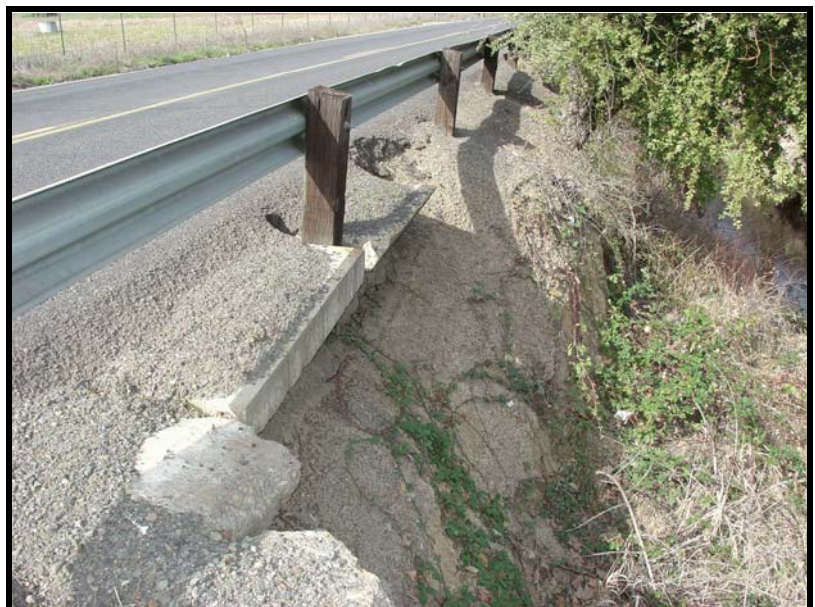
Existing Condition: Note severe erosion threatening stability of Grant Road.
