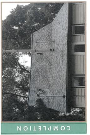
sheeting, shingles, flashing, ridge vents, and a moisture barrier. These completed repairs further the SCHT's This applicant and grant recipient's roof had been sagging and leaking for years. Previous attempts to fix these issues were not successful. With the assistance of a SCHT OOR grant, this applicant's roof finally received the necessary repairs. Hedrick Construction removed the existing roof and added new OSB goal of improving affordable housing in Story County,
