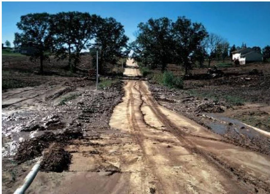
Figure 7D-1.01: Sediment in Street Due to Inadequate Erosion and Sediment Control During Construction
