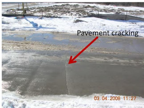
Figure 14B-2.07: Pavement Cracking Caused by HDD Installation
