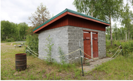
Vault toilet - park shelter area
