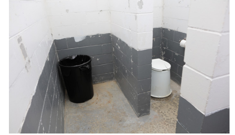
Vault toilet interior
