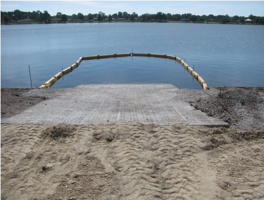
New boat ramp at Lake August; completion date is early January 2014.
