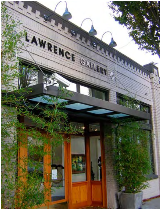
Recessed entry bay, protective canopy, transom windows, and decorative lighting
