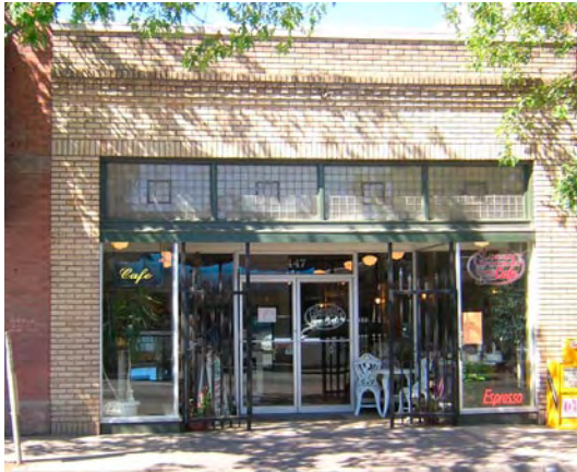
Large, recessed glass entry doors with flanking panels and transom windows creates an inviting building entry
