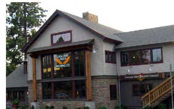
Wood columns and stone define the ground floor
