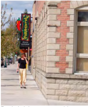
Basic brick masonry with quoins at the corner
