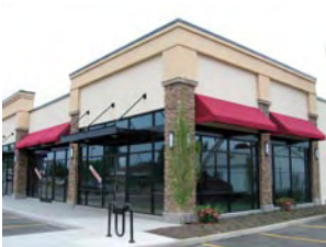
Stucco and stone
