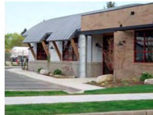
Brick, concrete, and metal
