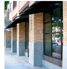
Canopies between architectural bays
