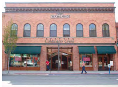
Recessed entry bay, protective canopies, engaged columns, and pedestrian-oriented signage
