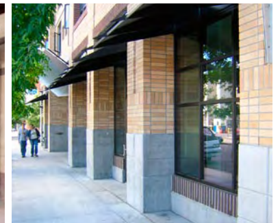
Plinths/columns and protective canopies
