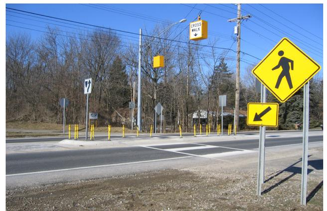
*This photo shows crossing treatments, including overhead and roadside signage, pavement markings, and a refuge island for a segment of the Clinton River Trail in Oakland County.*
