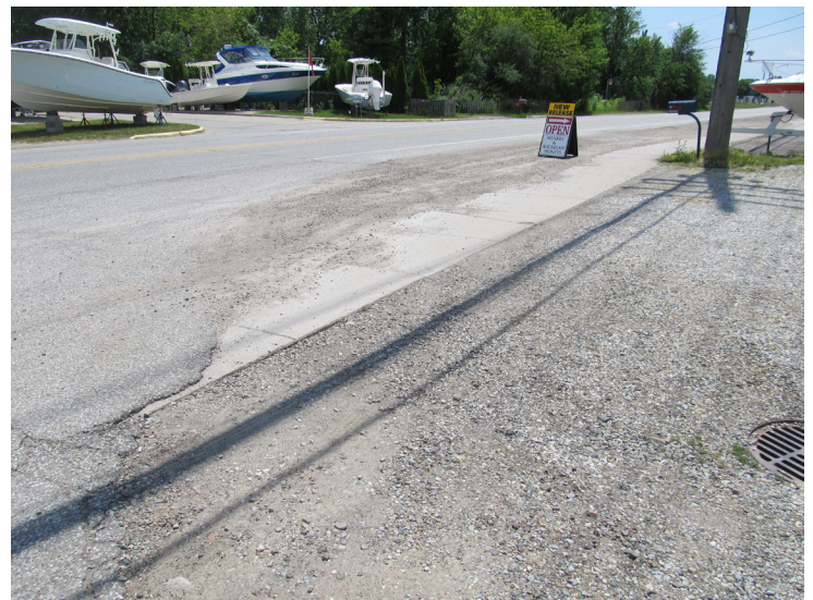
Location where the road, sidewalk and driveway are generally undefined.
