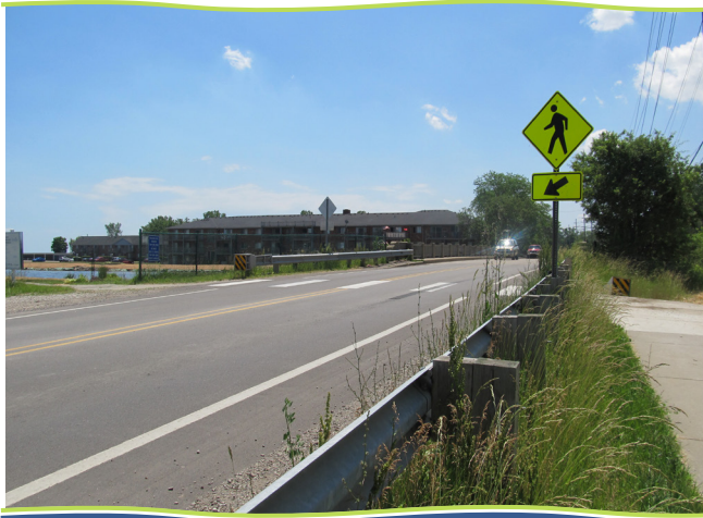
Jefferson Avenue approaching the Clinton River Spillway bridge
