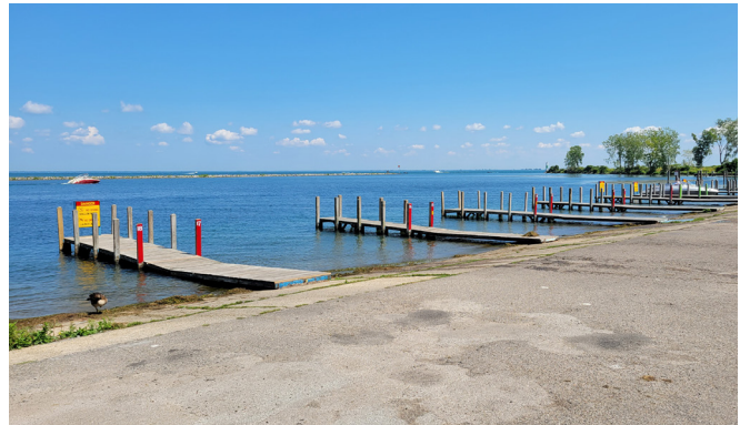
MDNR Boat Launch Site on South River Road
