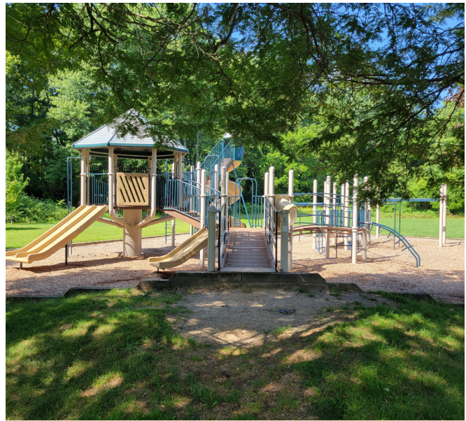
Example of a barrier-free obstruction to the playscape at Tucker Park
