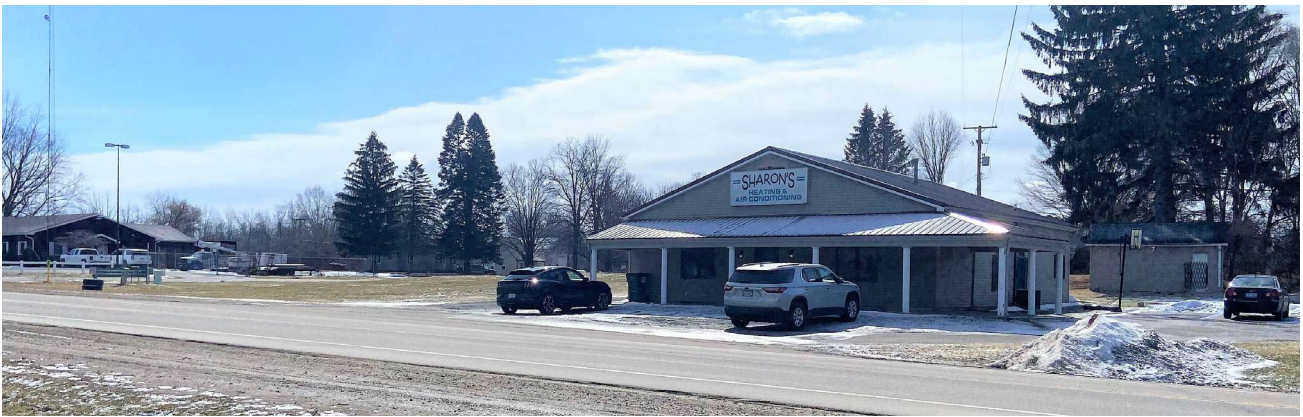
Figure 8: Sharon's Heating & Cooling, Mixed-Used Commercial District
