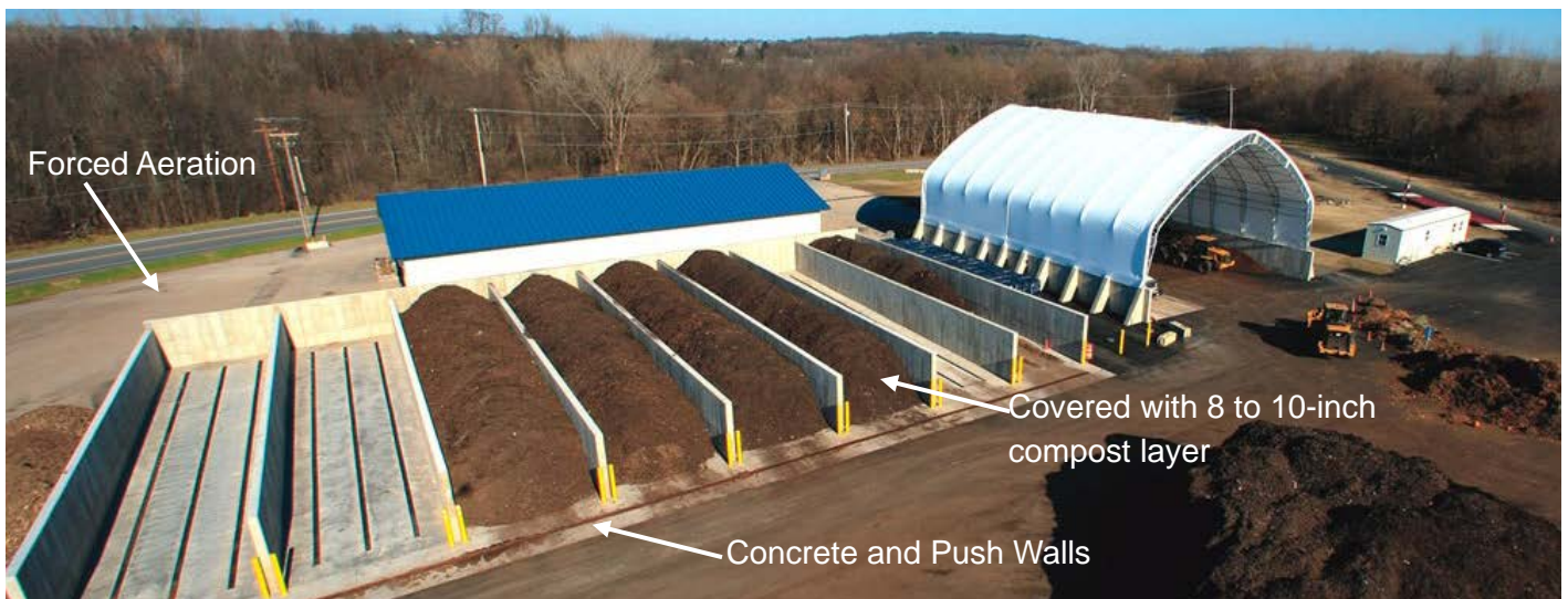
Photo Source: Onondaga Resource Recovery Authority, Syracuse NY (9,600 tons/year food scraps and 48,000 cubic yards/year yard trimmings)
