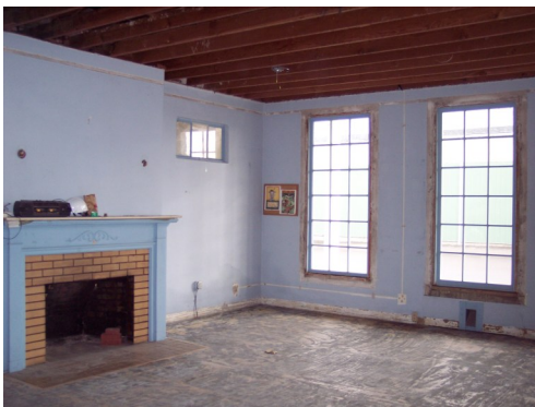
The Library Building Interior Early in the Renovation Process
