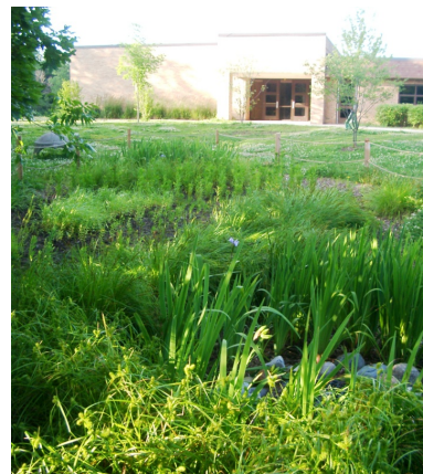
Figure 12. A rain garden captures water from the roof of a school in Ann Arbor, Mich.
