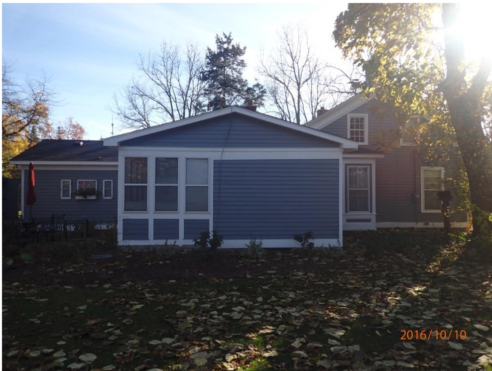
The north elevation with view of the summer kitchen porch addition
