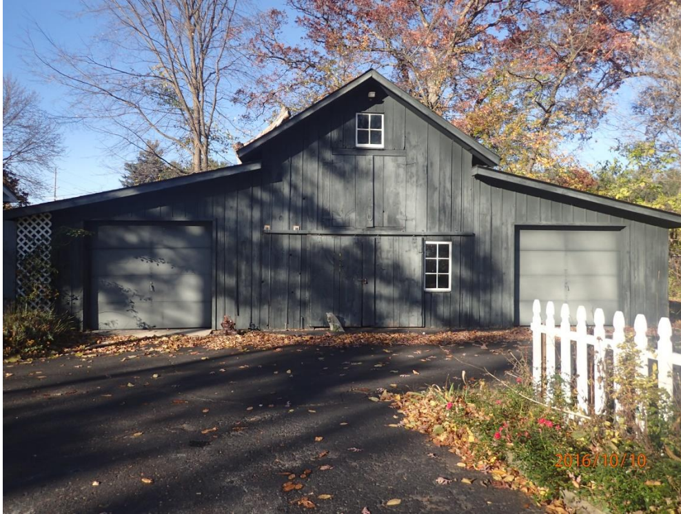
The south elevation of the c. 1876 carriage house and additions
