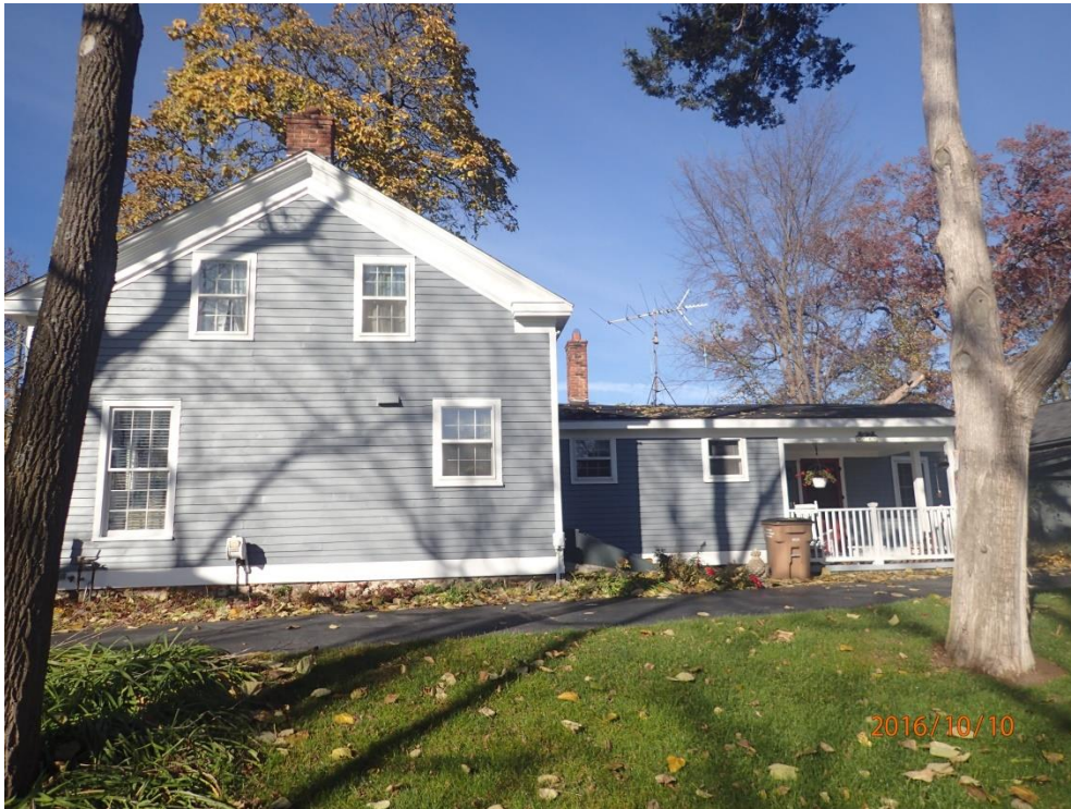
The south elevation of the Warden House with view of the 1890 addition
