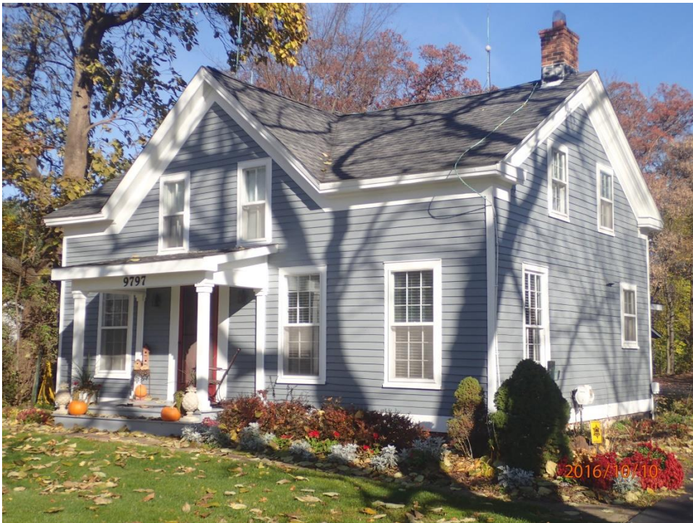
West (façade) and south elevations of the Warden House
