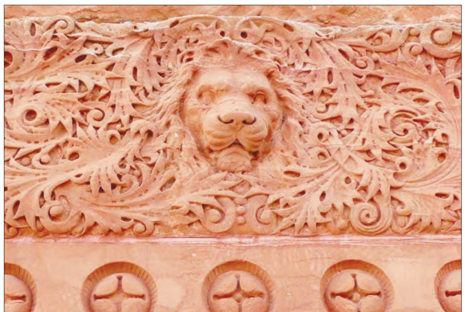
P.J. Glisson/The Globe INTRICATE DETAILS such as these are featured on the east side of the Gogebic County Courthouse in Bessemer. Historical data notes that red Jacobsville sandstone was used for the building. Streaked in white, the rock was quarried from a mountain a half mile away.
