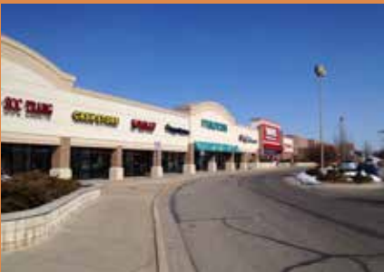
Commercial retail near Kalamazoo Ave. and South Beltline Highway
