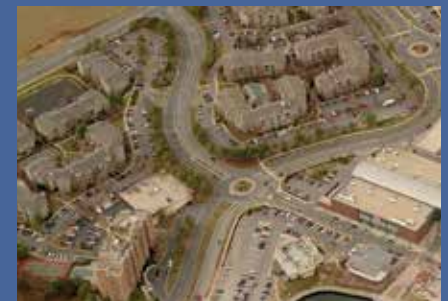
A mixed use development pattern is more likely to appear surrounding the M-6/M-37 interchange in the future
