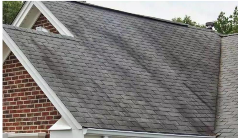
Typical staining from algae build-up
