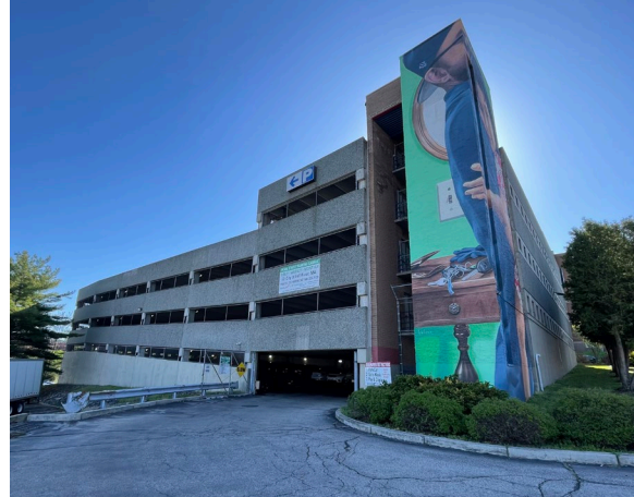
Figure 3 Pearl Street Parking Garage
