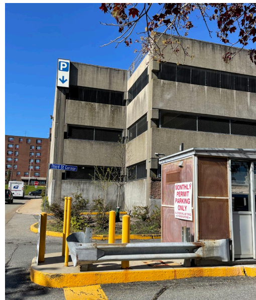
Figure 16 Third Street Parking Garage
