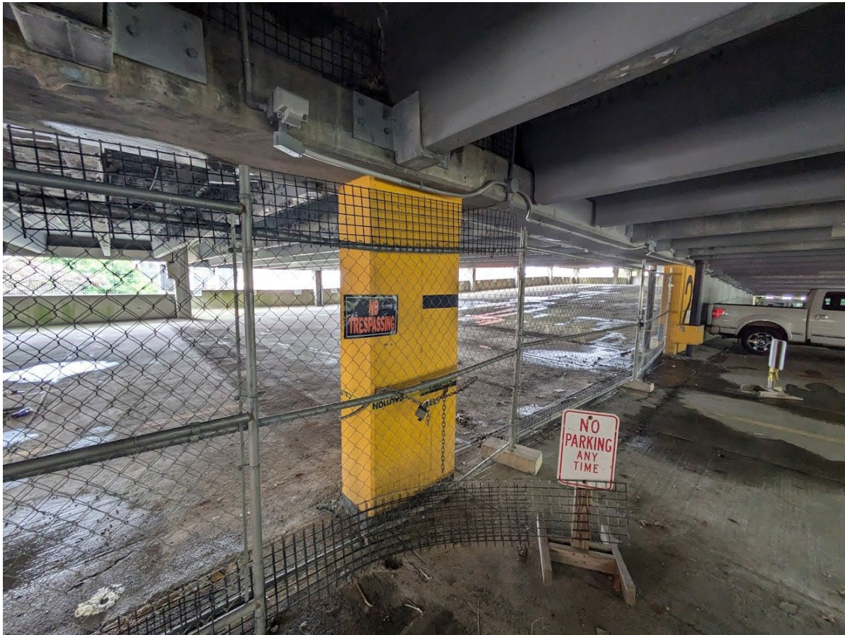
Figure 19 Level Closure at Third Street Parking Garage
