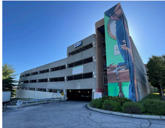
Figure 4 Pearl Street Parking Garage
