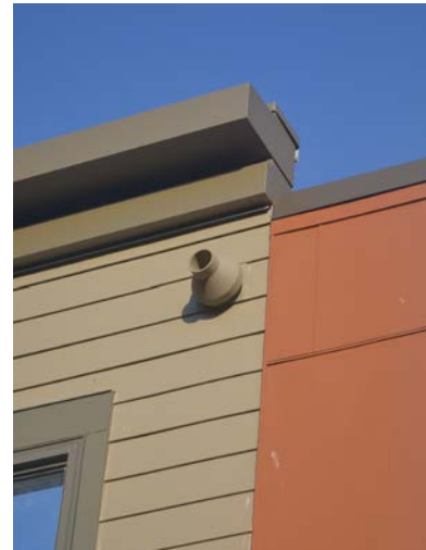
Exhaust vents and other mechanical attachments should match the façade.
