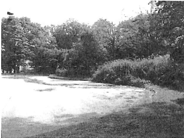
The historic wading pool. A drainage failure, originating at the comfort station (right of photo), created the wetland area on the east side of the pool.
