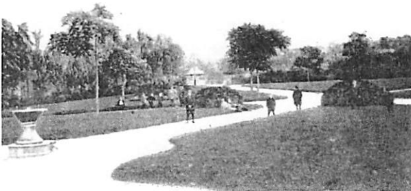
A series of broad concrete walkways, punctuated with trees and ornamental planting beds, replaced the original North Main Street entry, designed as a "music court" by the Olmsted Brothers. Postcard courtesy of the Fall River Historical Society.
