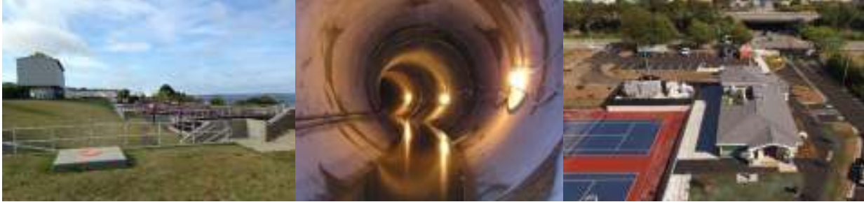
The upgraded Primary Treatment Facility and Sodium Hypochlorite Storage Facility at the WWTF (left). The CSO tunnel, bored through solid rock, toward the end of its construction (center). The recently completed President Avenue CSO screening and disinfection facility at Veterans Memorial Bicentennial Park (right).
