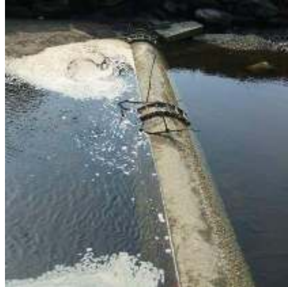
The exposed 36-inch Main Interceptor crossing within the open Quequechan River.
