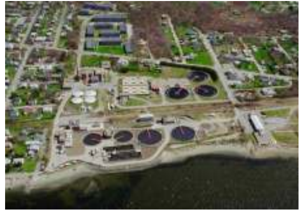
The Fall River WWTF is located at 1979 Bay Street.
