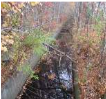
Open channel section of the existing North Watuppa Pond Interceptor Drain.
