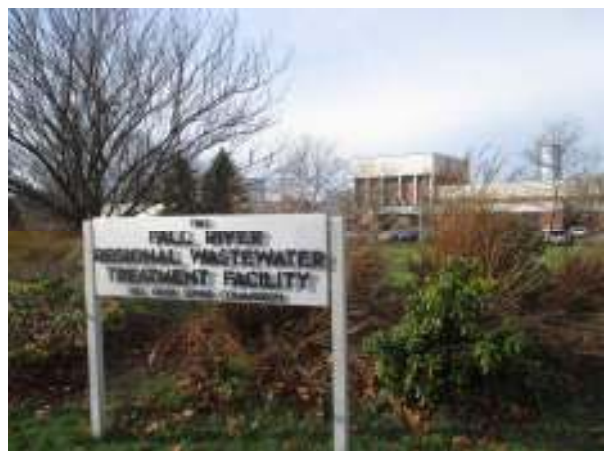
All wastewater and stormwater operations are based from the Fall River WWTF on Bay Street.
