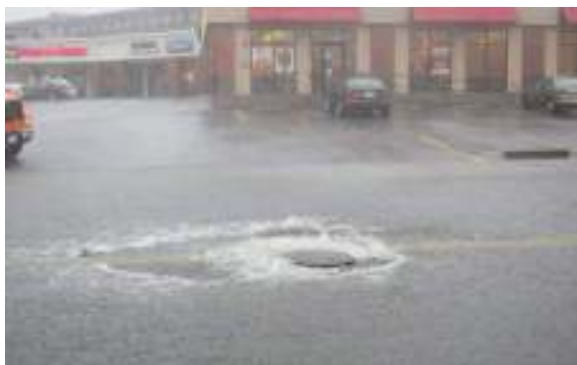
Sewer overflow due to insufficient pipe capacity in Stafford Square.
