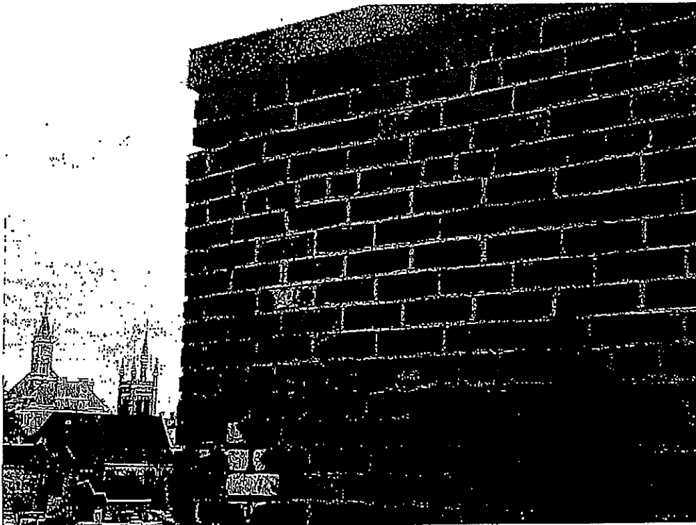
Exterior Masonry – re-pointing of existing joints required
