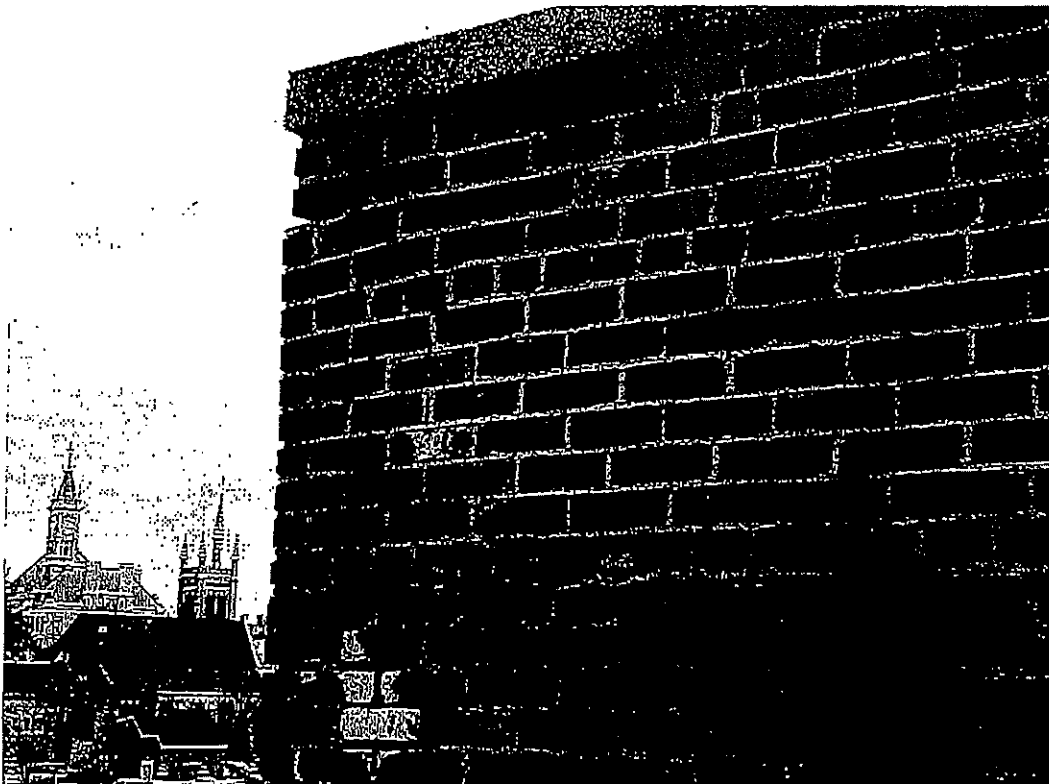
Exterior Masonry – re-pointing of existing joints required
