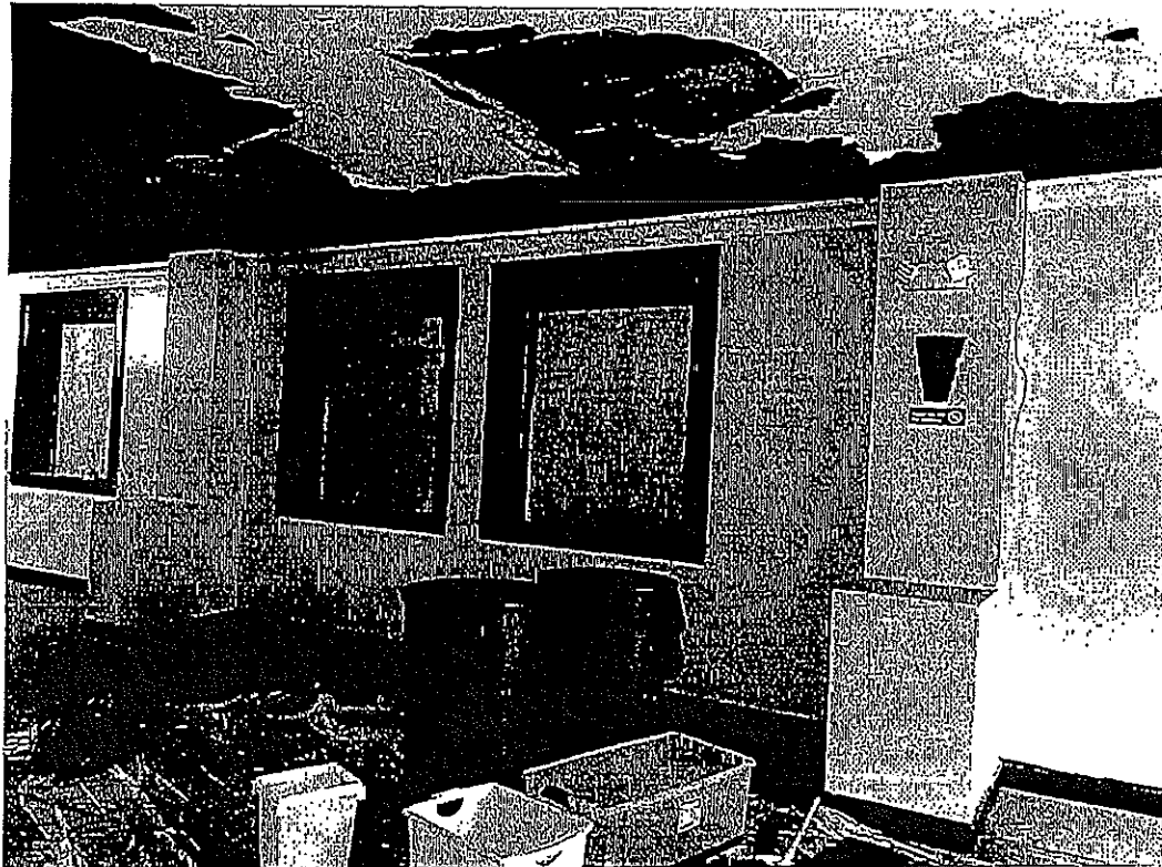
3 rd Floor – significant ceiling deterioration caused by water infiltration as a result roof system failure
