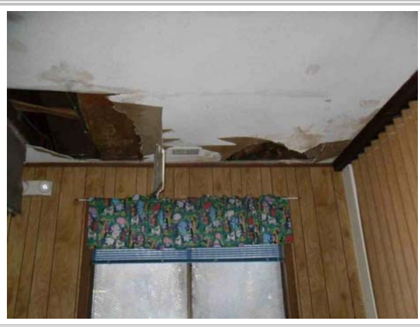
Ceiling Water Damage
