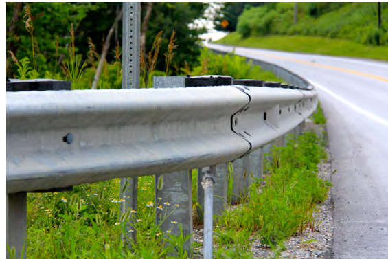
W-beam guardrail on east side of Route 104 constricts bicyclists and pedestrians to a narrow shoulder.
