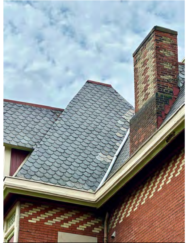
Photo 4. William & Mary Spencer House, Primary Façade facing South West, M. Falcone. February, 2026.
