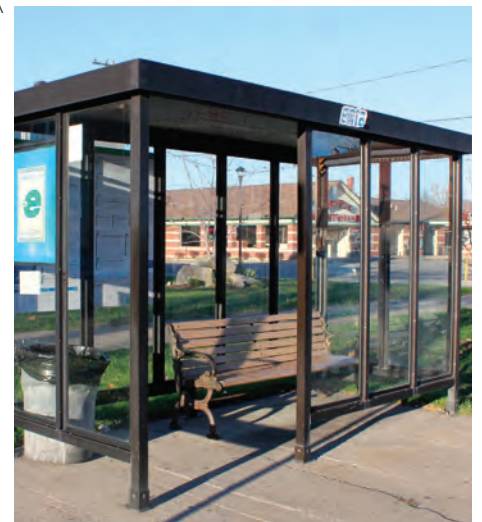
Existing EMTA bus shelter
