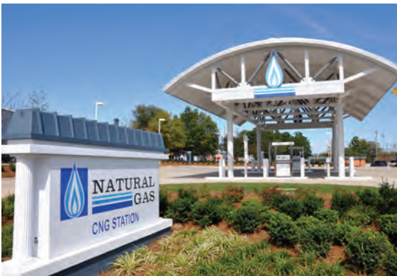
Example of CNG gas station
