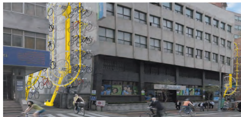
Potential bike storage facility
