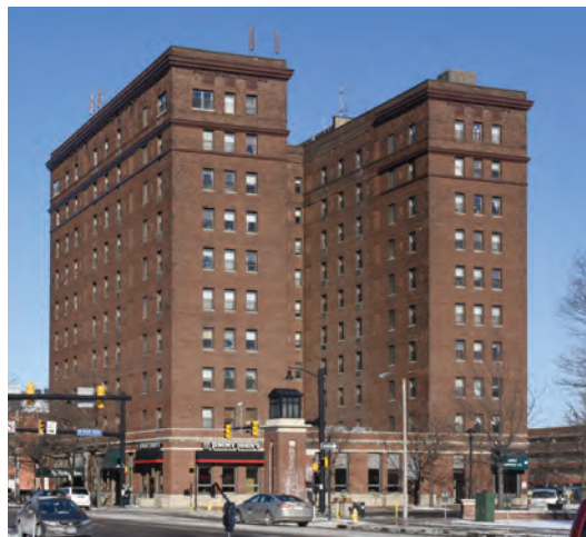
Existing residential building in downtown
