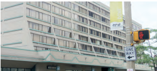
Existing hotel today
