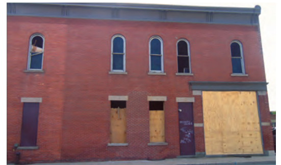
Renovations on the Turnpike building
