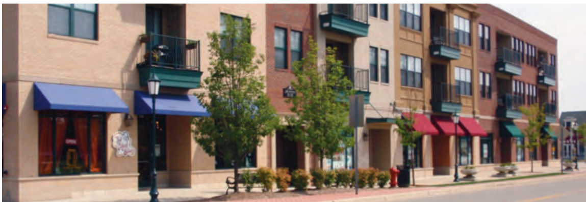
Example of successful building wall articulation
