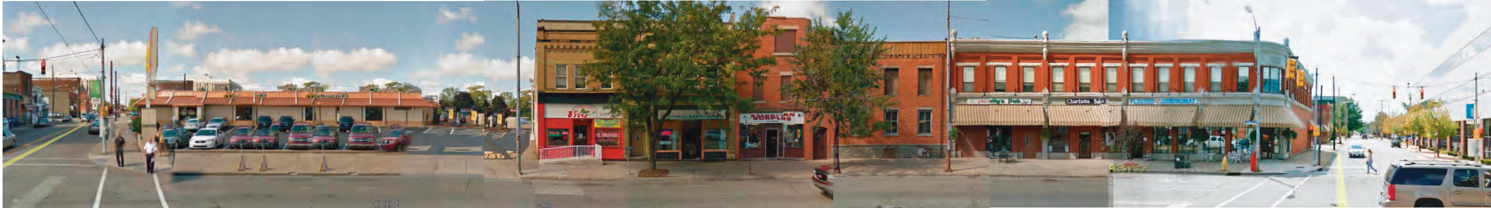
Example of Priority Buildings (State Street between 4th and 5th Streets)--Before
