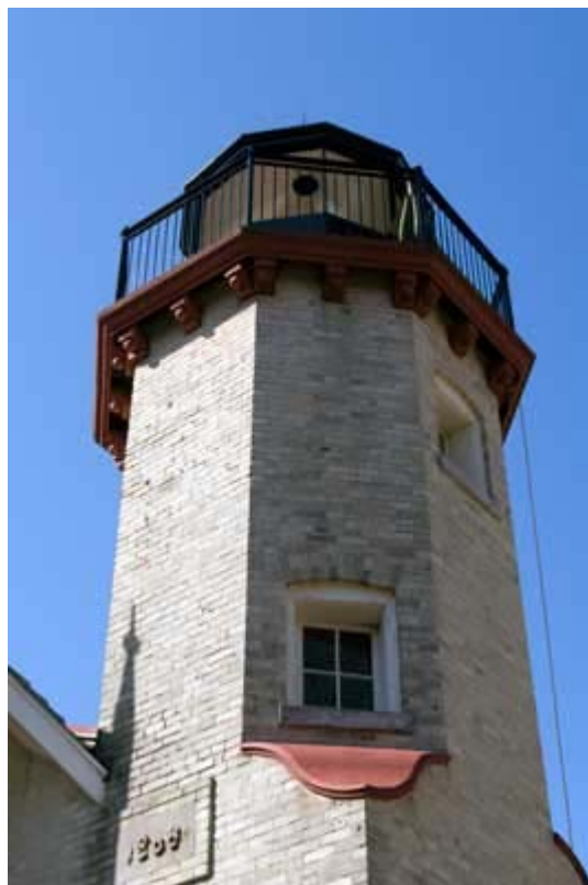
Completed Tower with Lantern and Railing the Next Day (Friday)
