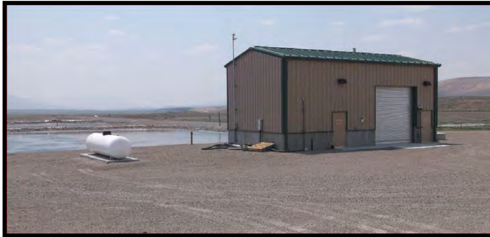
Waste Water Treatment Facility
