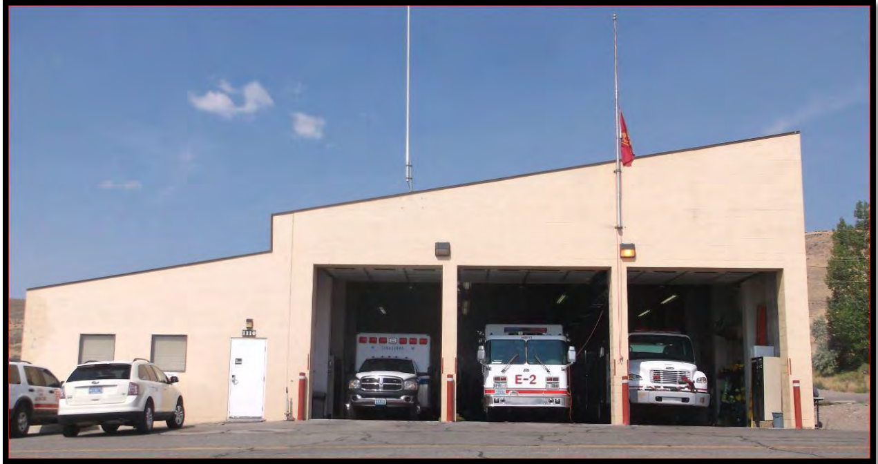
Jackpot Fire Protection Facility
