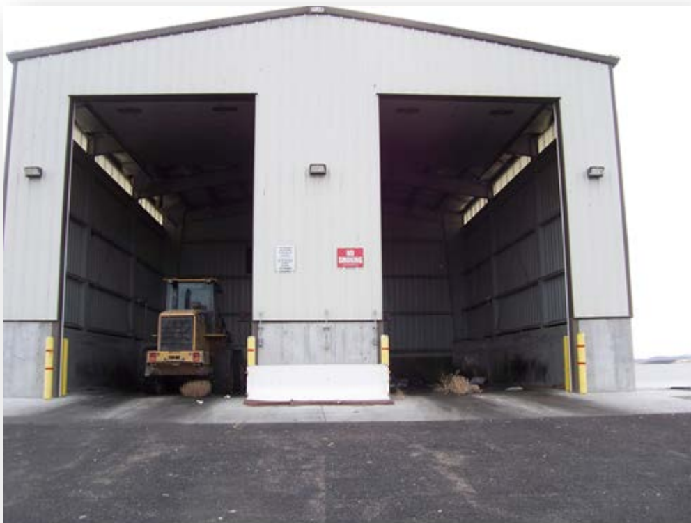
Figure 4: Elko County constructed and owned transfer station at Jackpot
