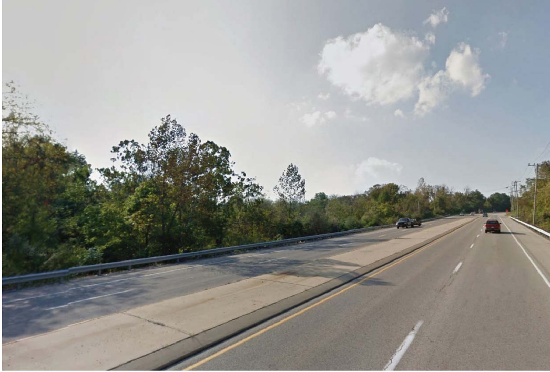
GREAT VALLEY CORPORATE CENTER: PHOTO LOCATION VIEW 7
