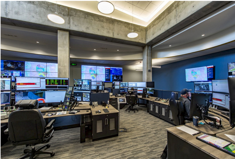
Photo: Inside the SEMRECC 911 Dispatch Center
