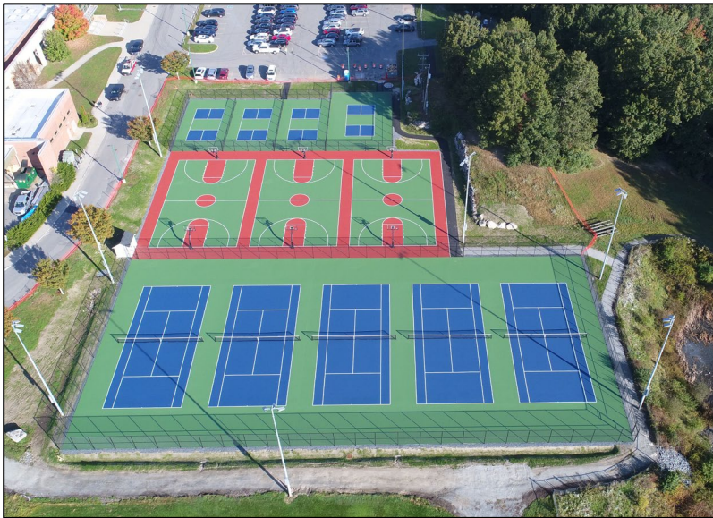
Above: New courts at Oliver Ames High School
