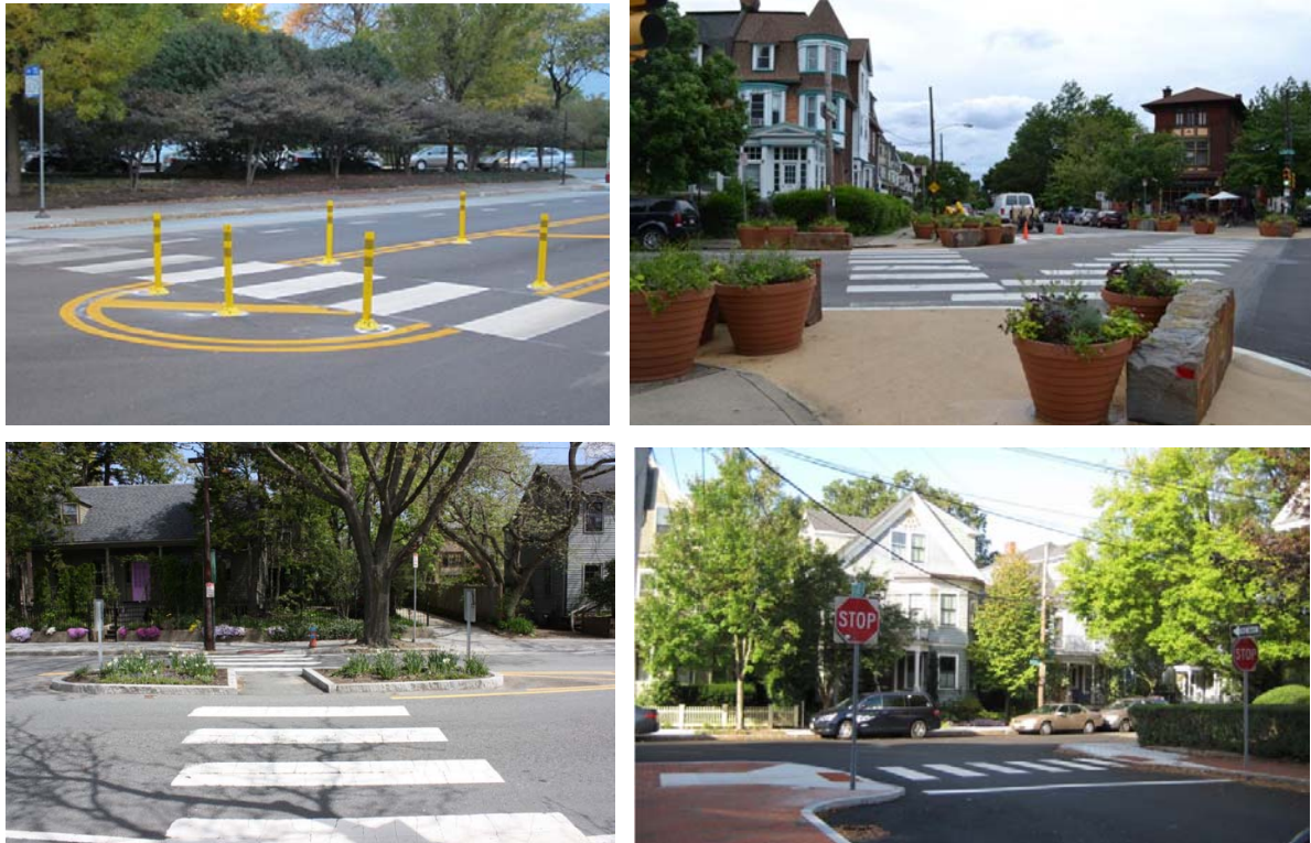
(clockwise from top left: interim median crossing island with paint and bollards; interim curb extension with paint and planters; permanent curb extension on side street; permanent median island with landscaping)
