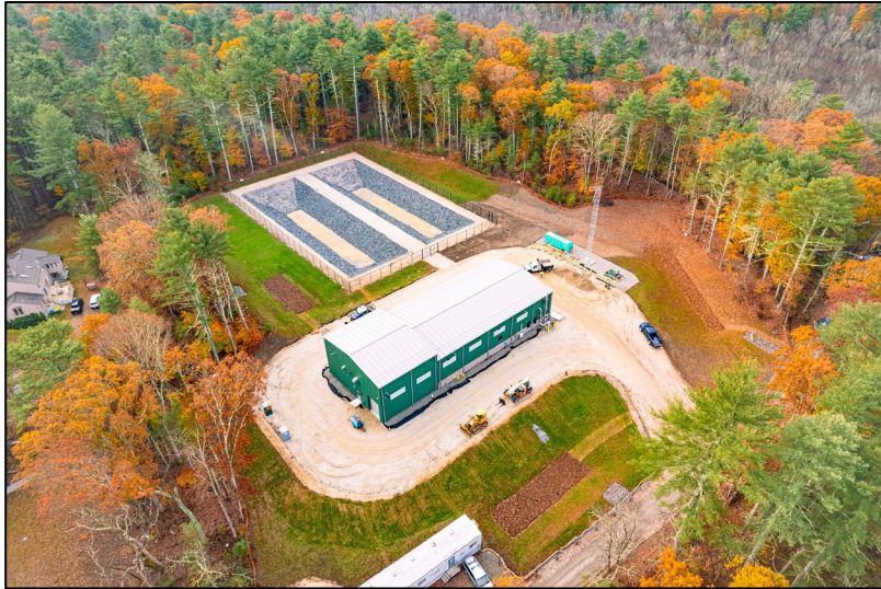
Above: Red Mill Road Treatment Plant
