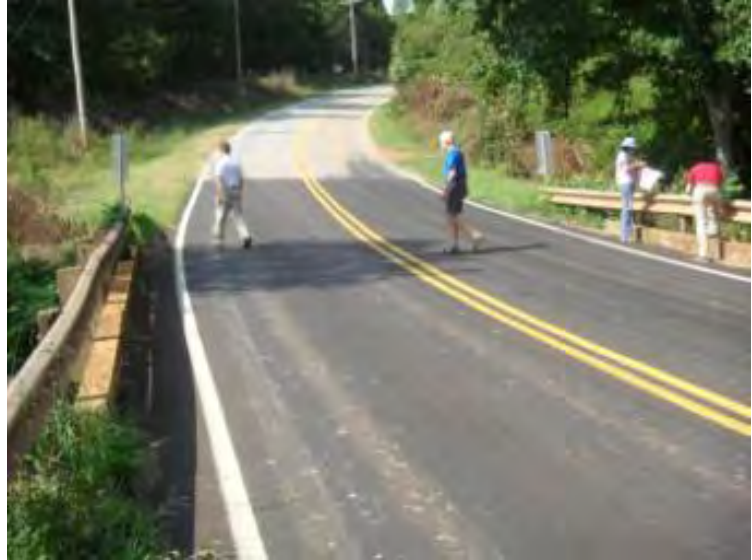
Pearson Road bridge over Brushy Creek. Pearson Road has potential site-distance issues for trail crossing due to the curve west of the creek.
