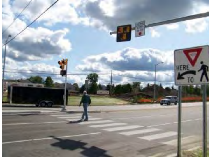
HAWK signal with high-visibility pedestrian crossing
