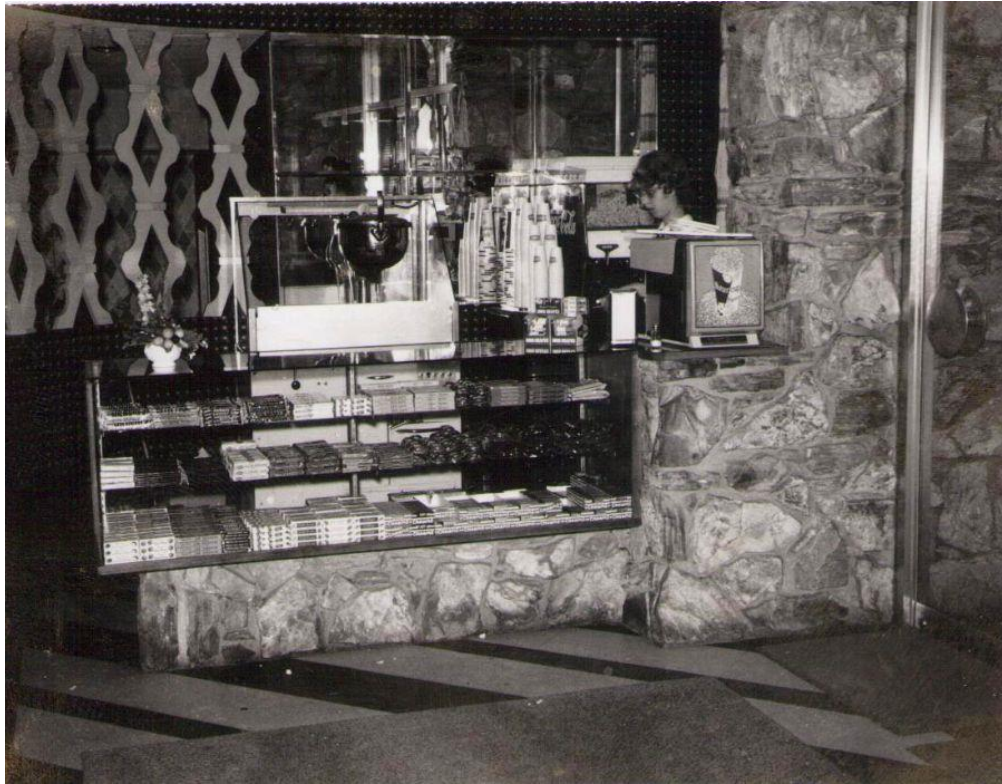
Figure 105: Lobby concession booth, looking south, October 1958 (Courtesy of Brian Fridley)
