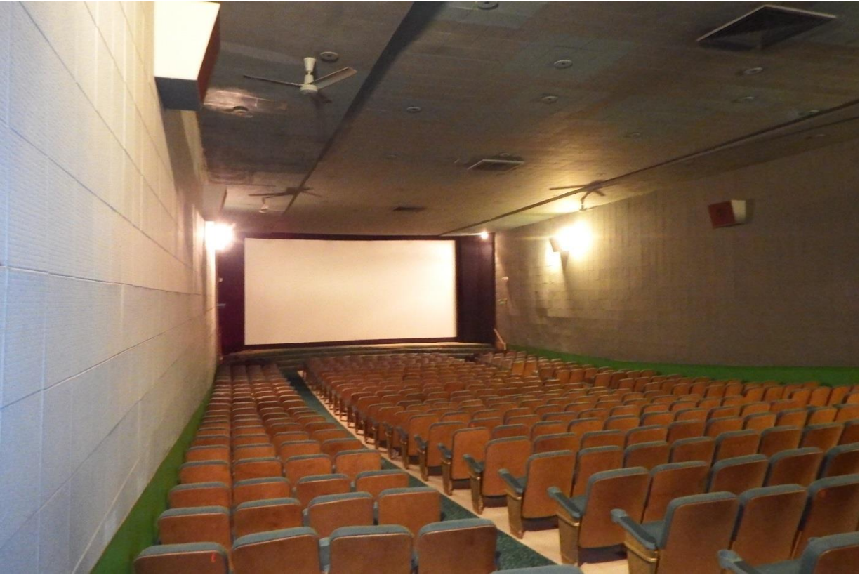
Figure 6: Current auditorium, looking southeast (Jacobsen, 2020)
