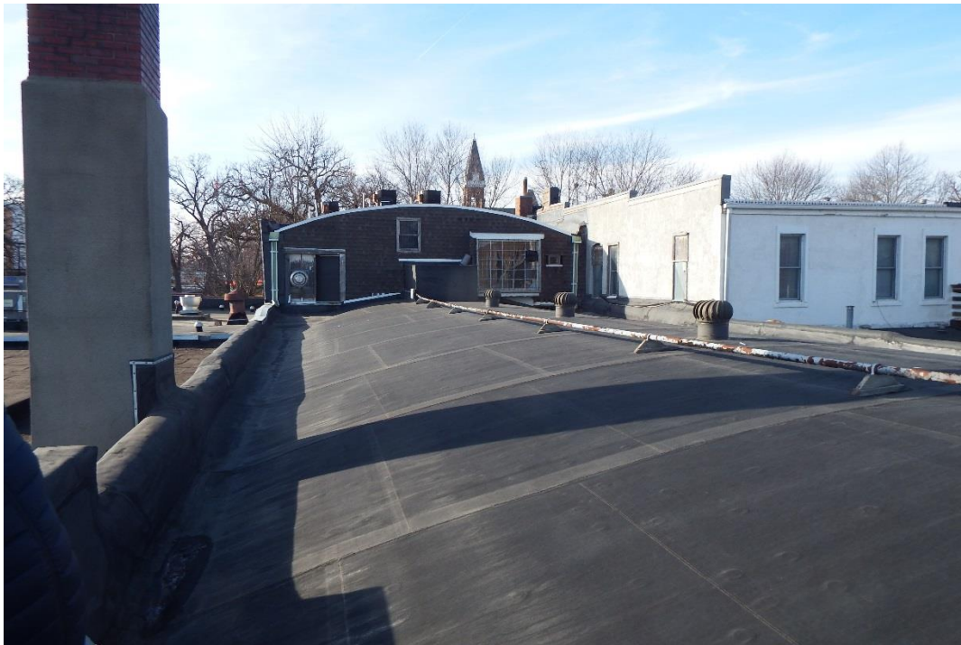
Figure 19: Current roof overview, looking northwest (Jacobsen, 2020)
