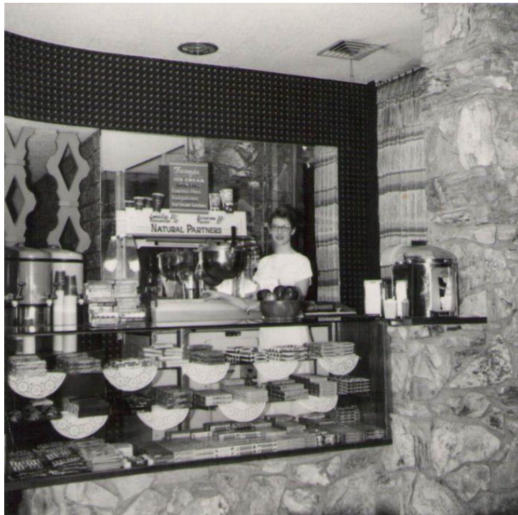
Figure 104: Lobby concession booth, looking southwest, October 1958 (Courtesy of Brian Fridley)
