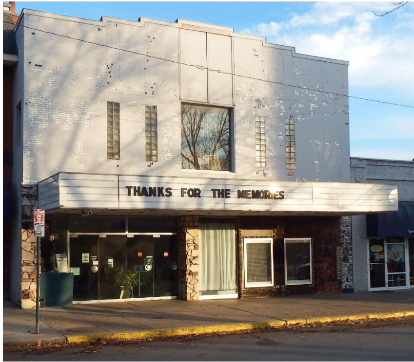
Figure 2: Current façade appearance looking southeast (Jacobsen, 2020)
