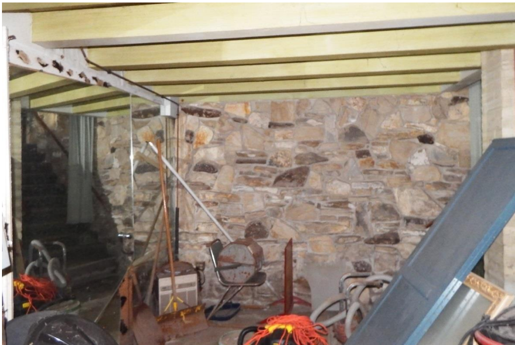
Figure 3: Current basement lobby looking north (Jacobsen, 2020)
