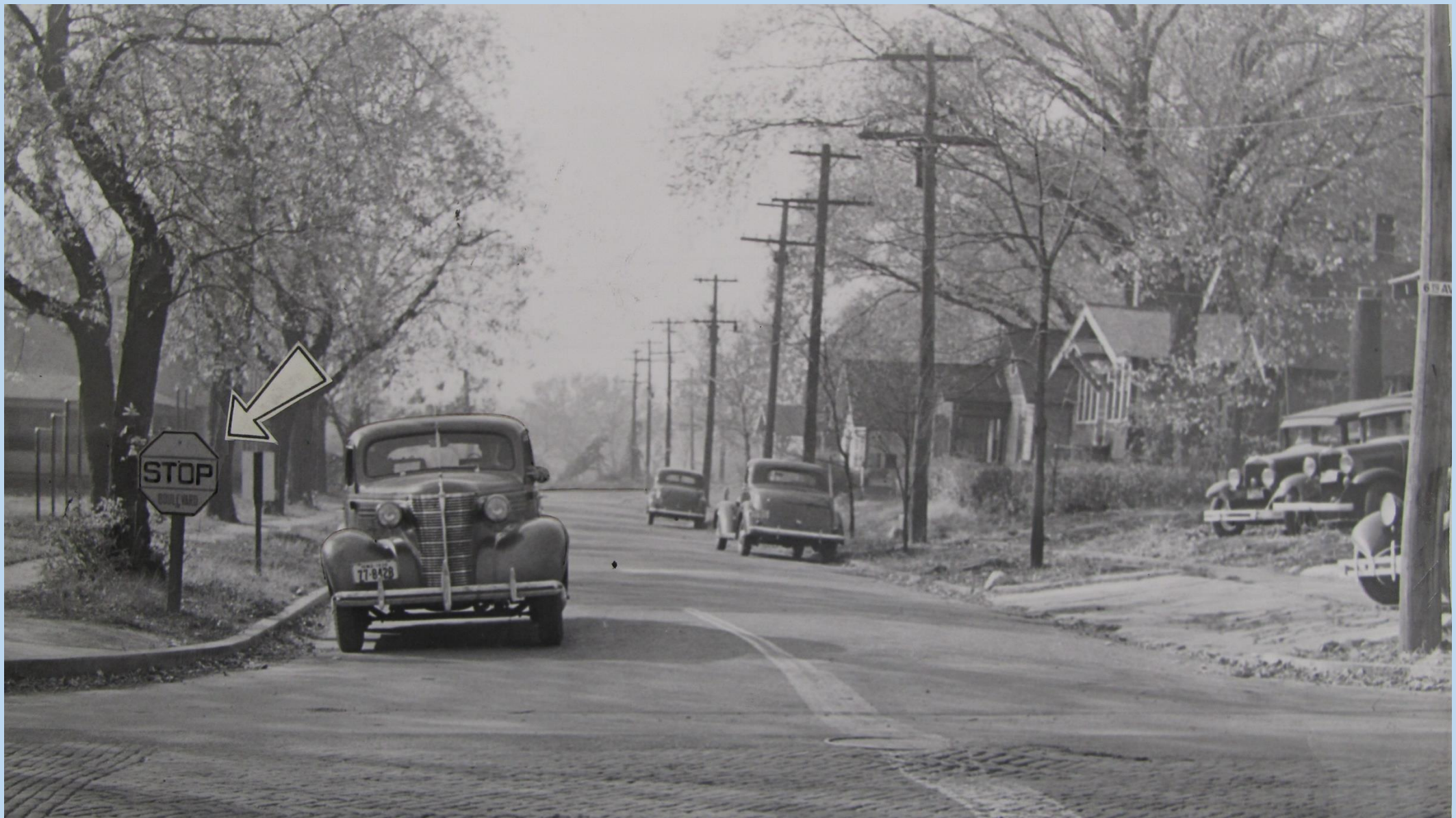
Undated: view down Boston from 6 th Ave. Is this STOP sign installed backwards?
