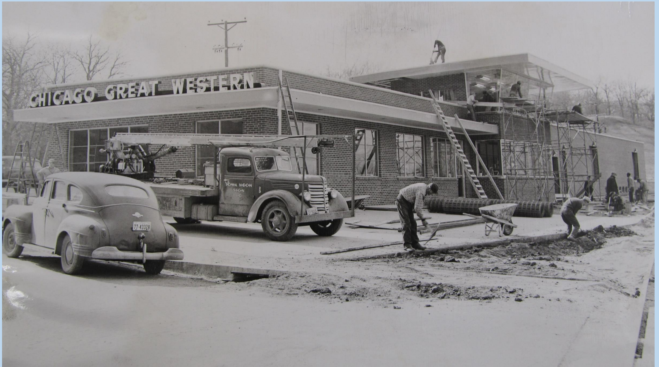
November 1950: Great Western Railway station under construction
