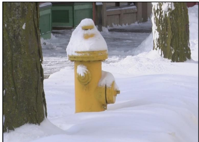
Figure 2. Tree and hydrant compatibility require proper distancing
