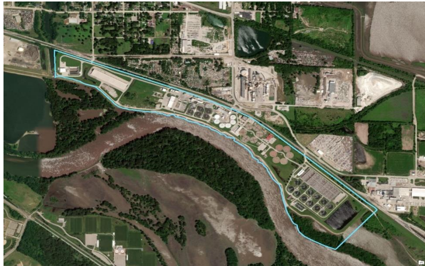
Figure 5. WRA facility at 3000 Vandalia Road on the east side.
