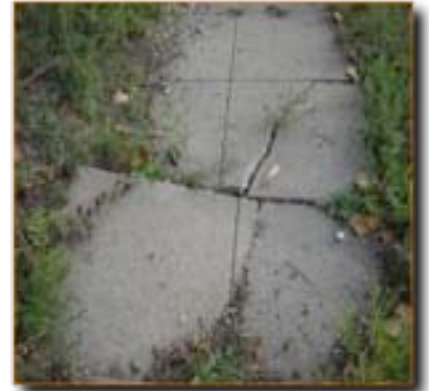
Figure 13. Cracked sidewalk
