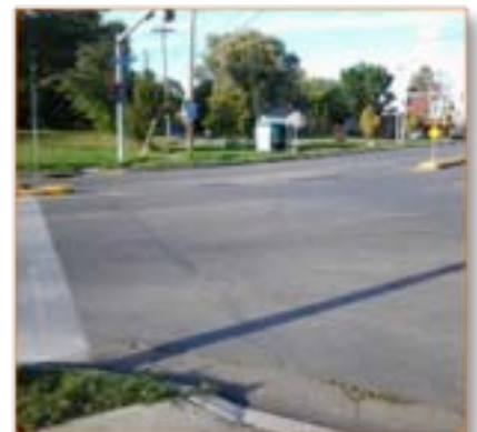
Figure 16. No sidewalk infrastructure
