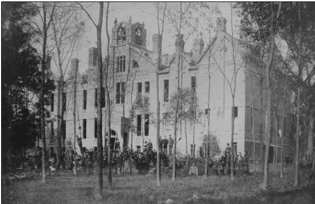
Figure 3-1: The construction of Old Main, view northeast, 1882 (Quax, 1906)
