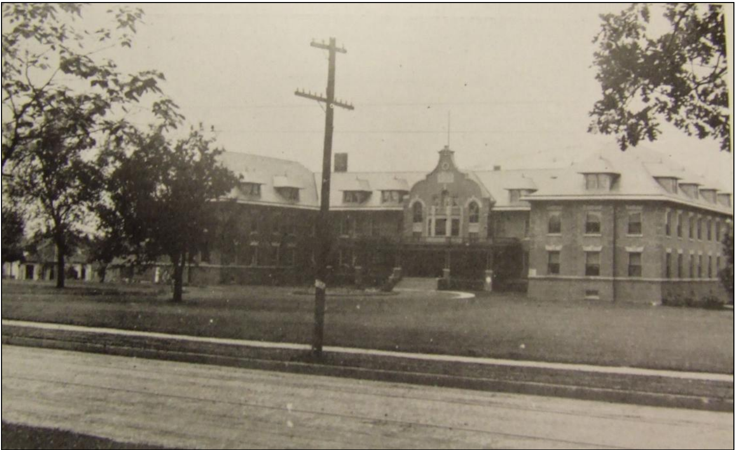
Figure 3-26: Home for the Aged, view northwest (Quax, 1908)
