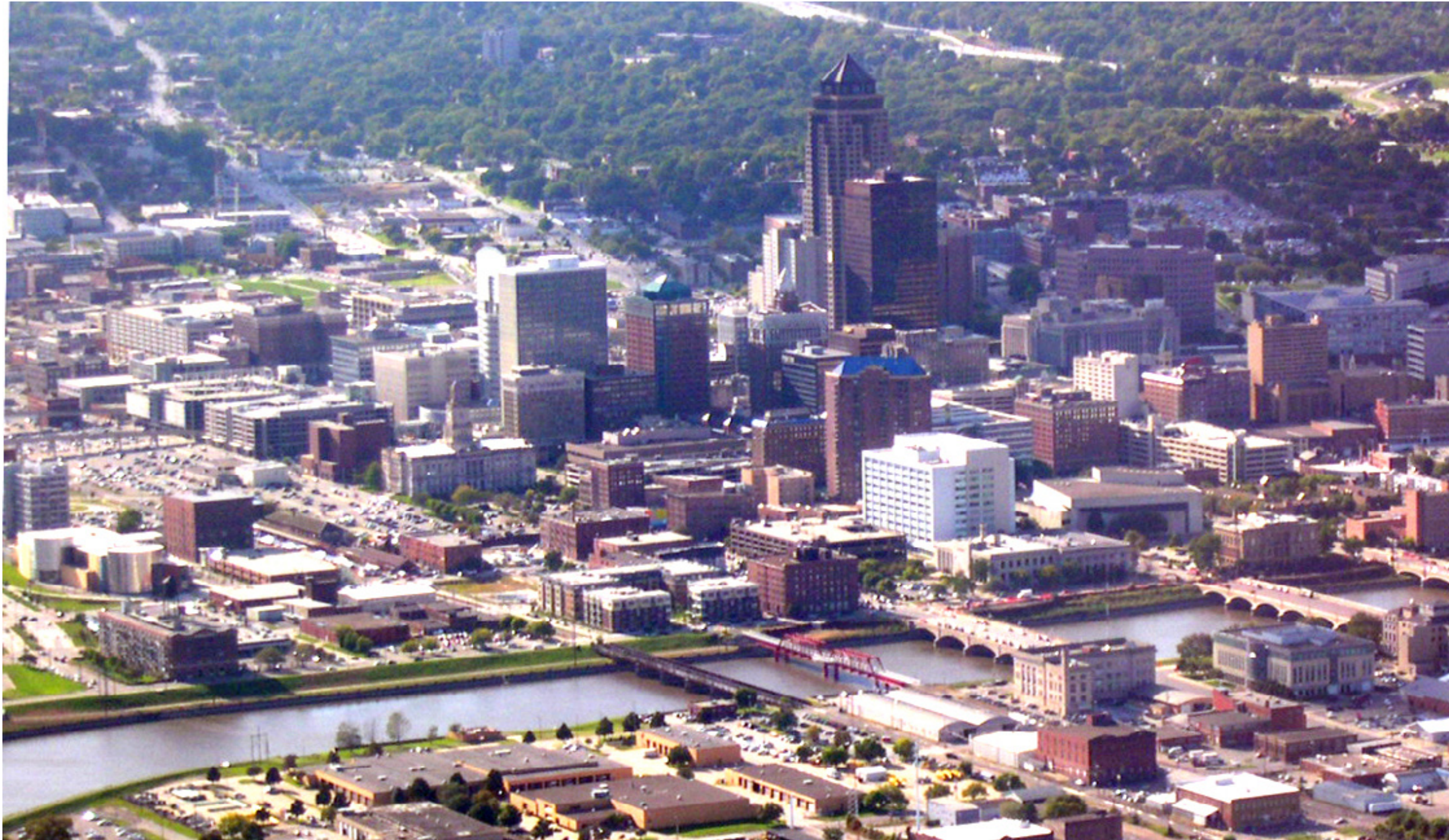
aerial photograph of downtown looking northwest: Des Moines River and downtown Des Moines skyline, September 2006
