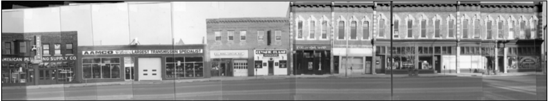
North side of Grand Avenue between East 5th and 6th Streets: an excellent example of the beginning of block rehabilitation
