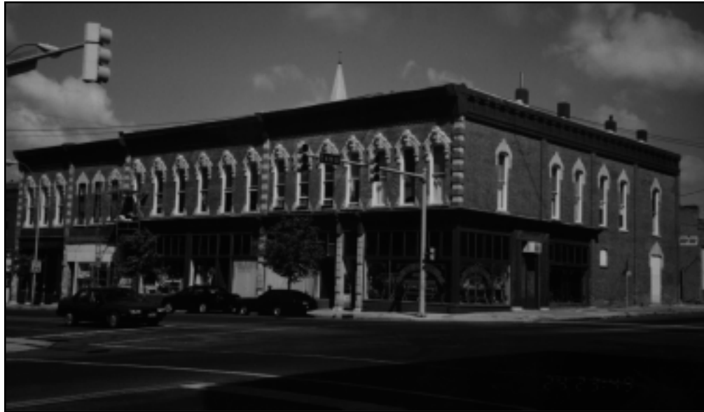
506 to 526 East Grand Avenue: an inspirational example of building rehabilitation that provides spaces for housing, live/work and retail
