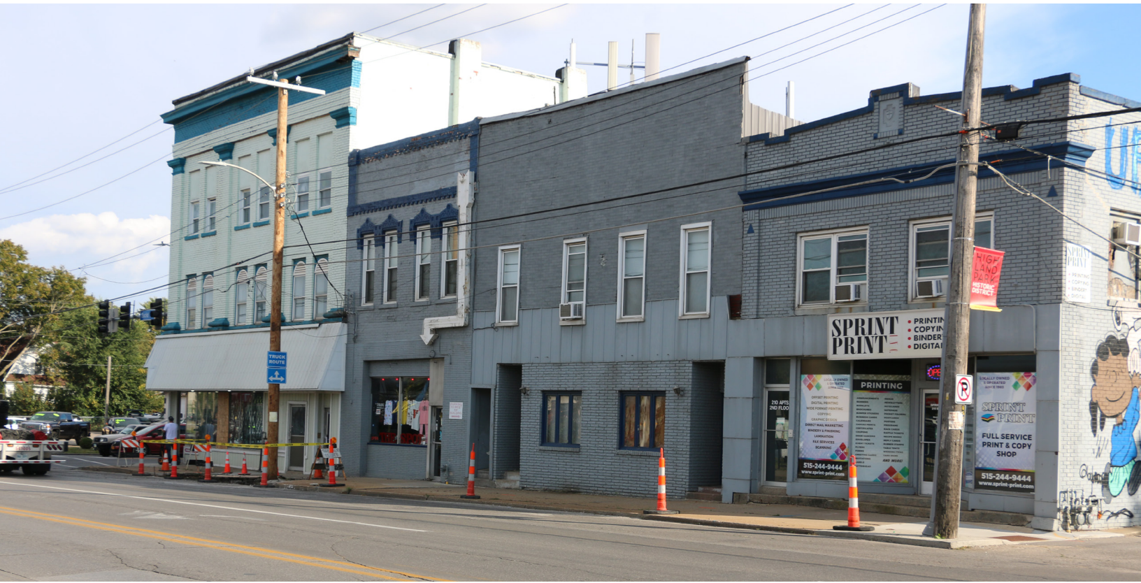
200 Euclid Avenue Exterior | Looking southwest (top) + southeast (bottom)
