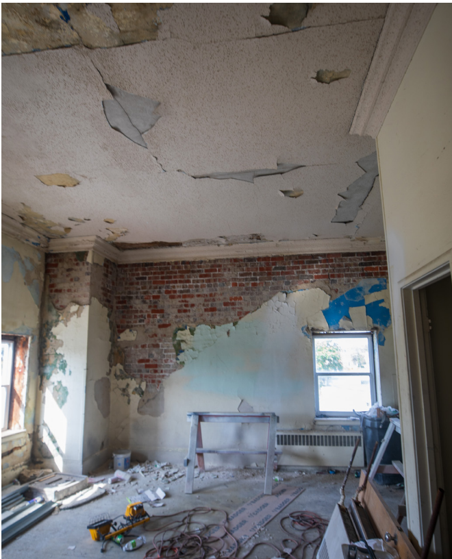
200 Euclid Avenue Interior | Second Floor
