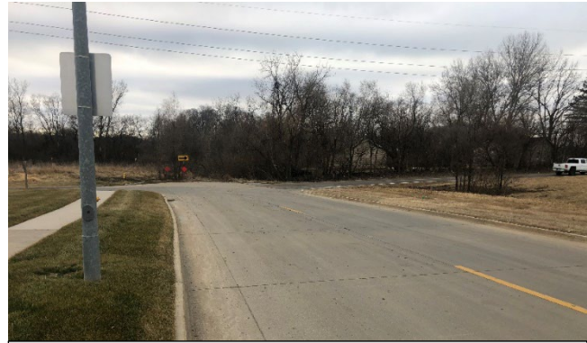
A future realignment of SW 56th Street is needed to connect with previously improved alignment to Park Avenue.
