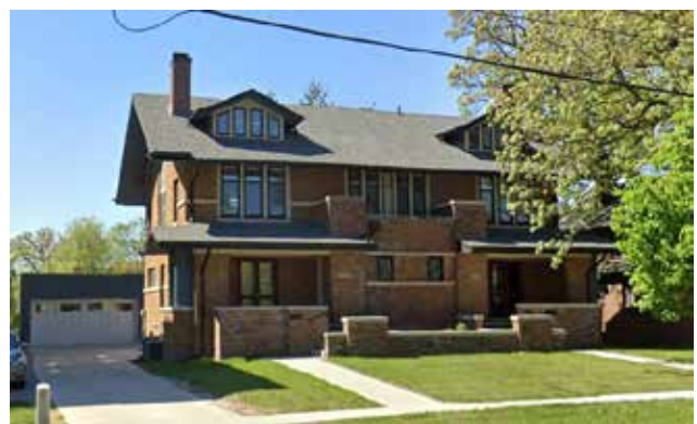
Figure 33. Stockdale Double House, a local landmark, is an example of a multi-unit historic structure. (Source: Google Earth)
