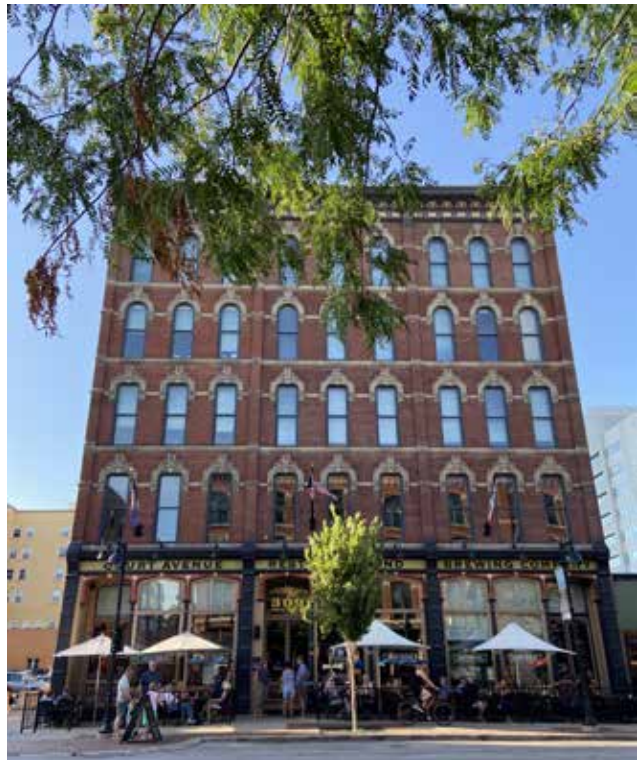
Figure 13. Saddlery Building, 309 Court Avenue (Source: Stacey Hanley)
