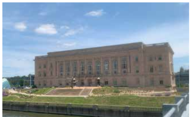
Figure 25. Des Moines City Hall (Source: KKC)
