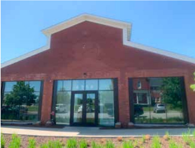
Figure 28. 6908 Chaffee Road, a building on the Fort Des Moines campus that has been rehabilitated and is in active use. (Source: KKC)
