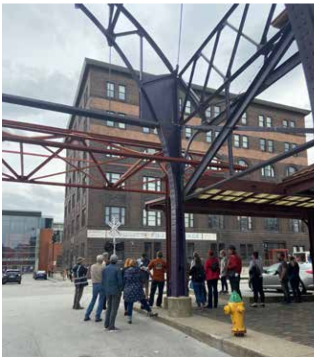
Figures 7 and 8. Iowa Architectural Foundation Walking Tour. (Source: Stacey Hanley)
