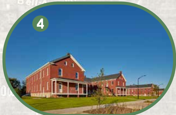
Figure 15. Fort Des Moines (Source: Architect Magazine)
