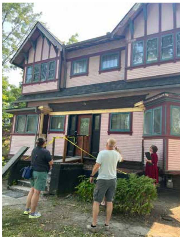
Figure 13. Site meeting with two HPC members and a contractor to discuss an in-progress project in the River Bend neighborhood. (Source: Stacey Hanley)
