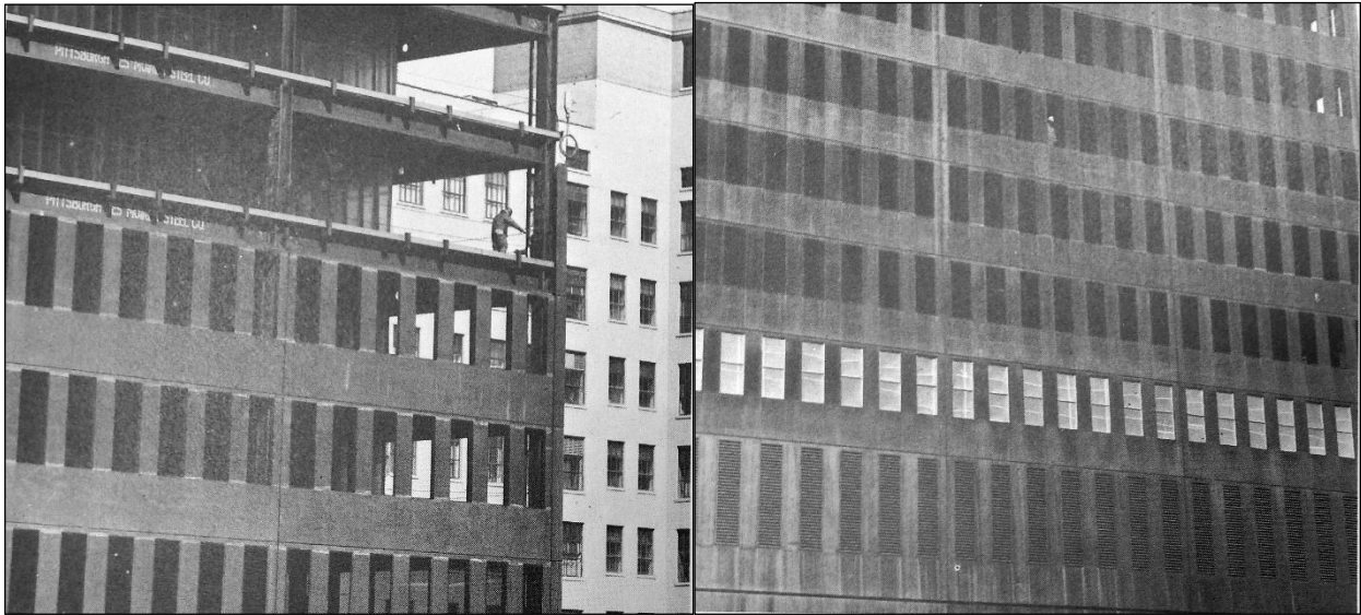
Figure 64: Left, note mounts for wall panels, right, temporary window coverings (Structural Report)
