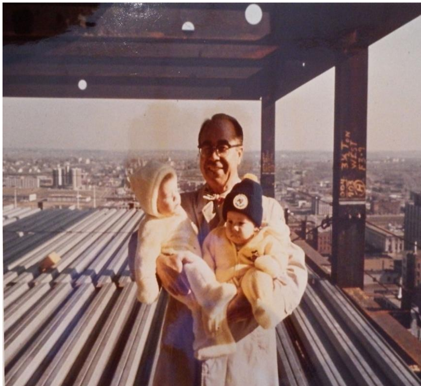
Figure 28: John Ruan and grandchildren, looking east, 1974 (note steel forms for concrete floors and the vertical column splices) (Ruan Scrapbooks)
