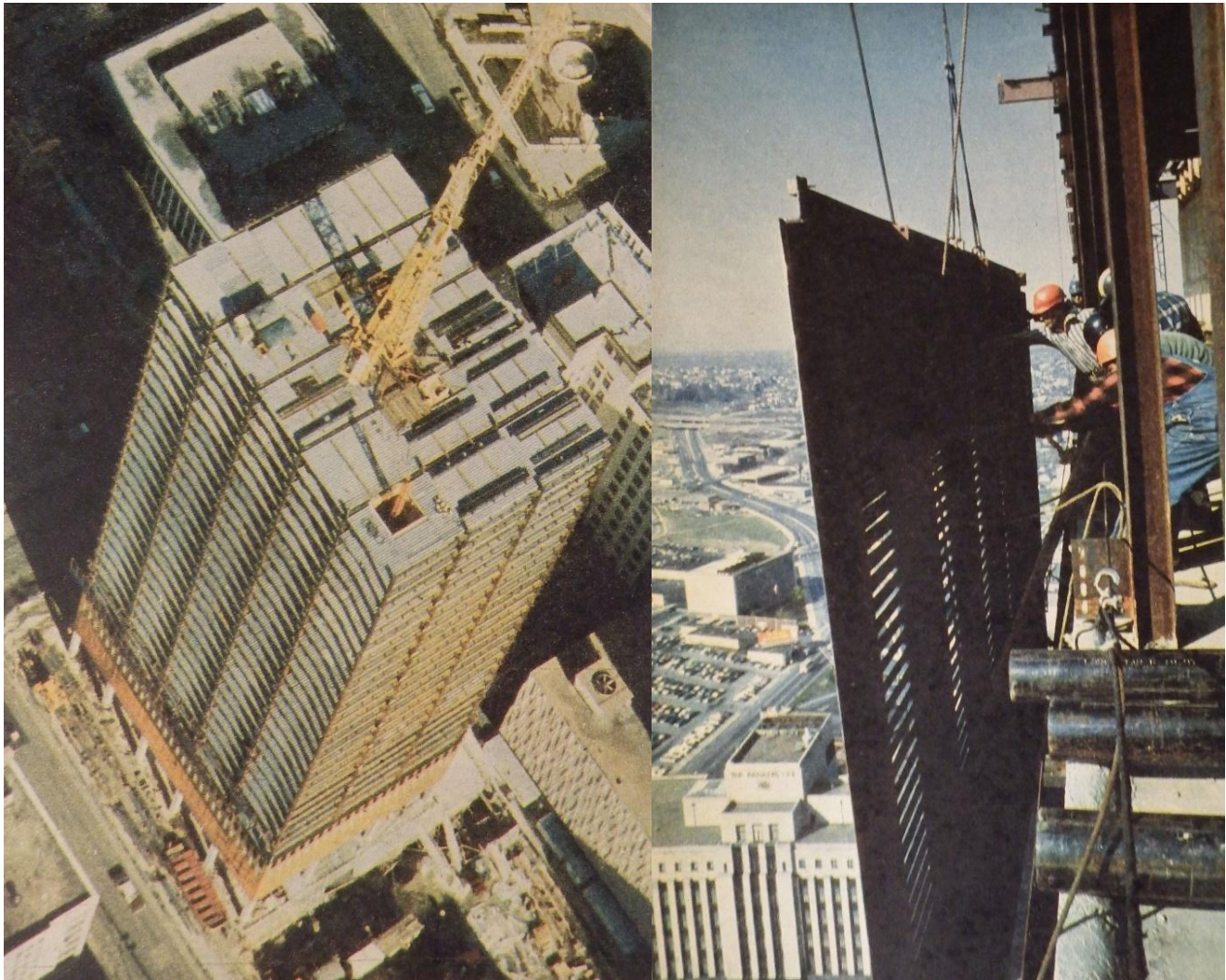
Figure 66a: Left, aerial view looking northeast. Figure 66b: Right, lifting a top floor louvered curtain wall panel, looking north (note the temporary freight elevator inset in the southwest corner) (Des Moines Register , June 1, 1975)
