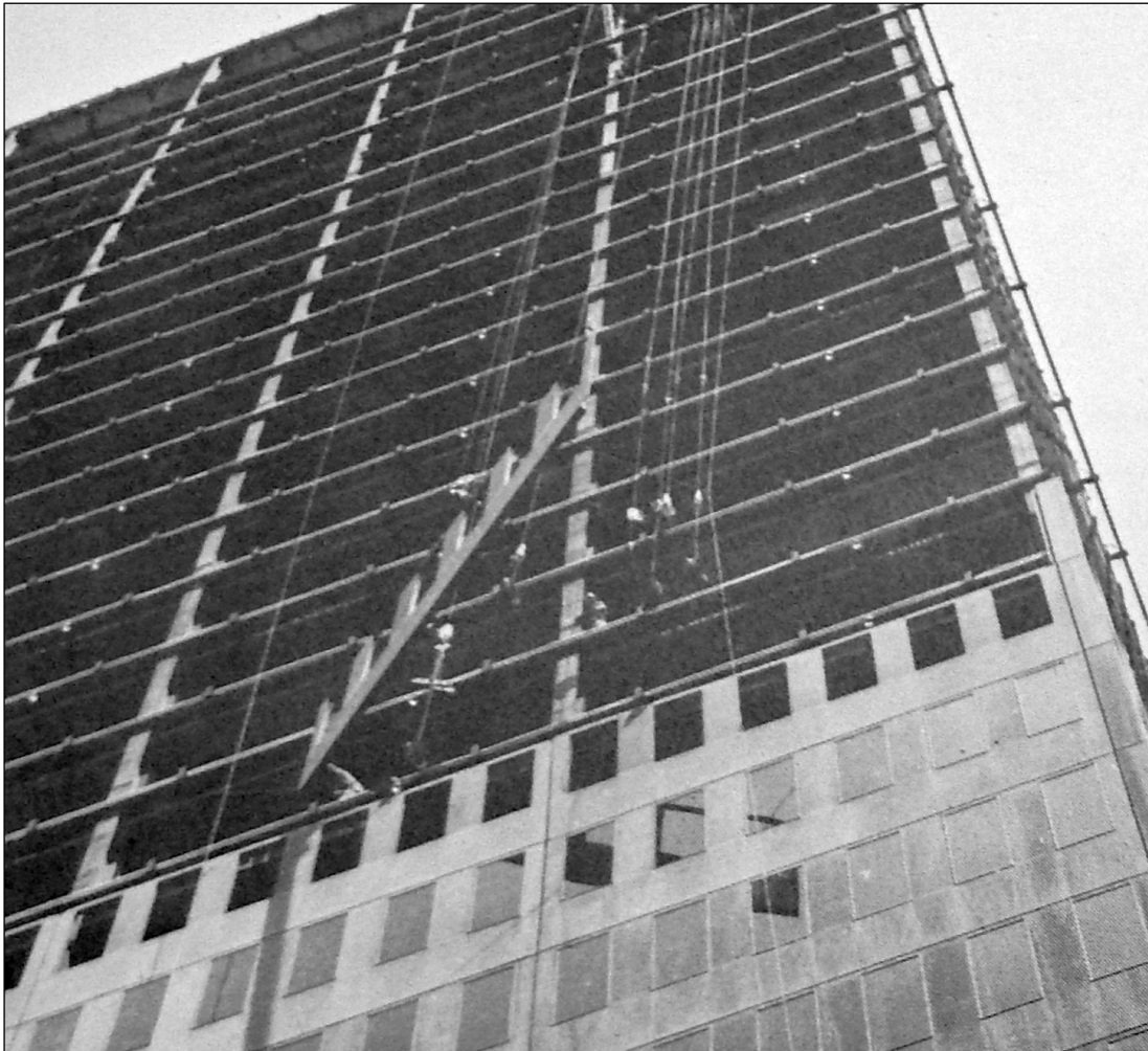
Figure 65: A wall panel is raised to the fourteenth floor, looking southeast (Structural Report)
