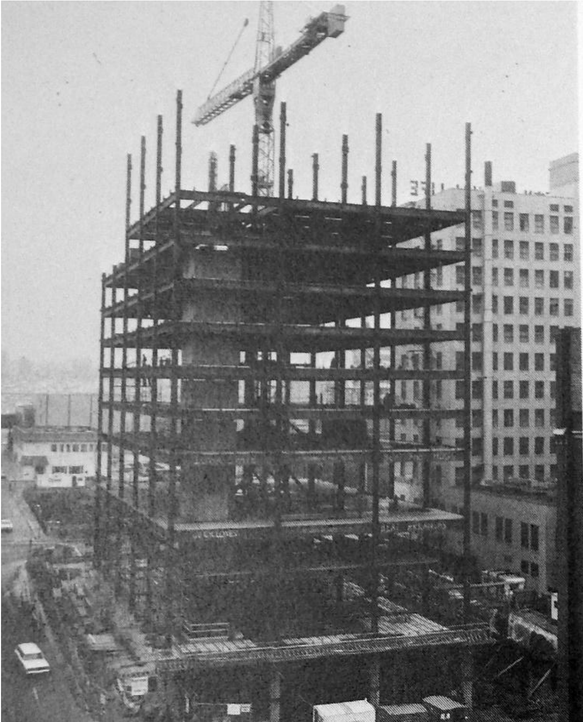
Figure 59: Construction progress, looking north showing temporary southwest corner elevator. (Structural Report “Ruan Archives”) 120
