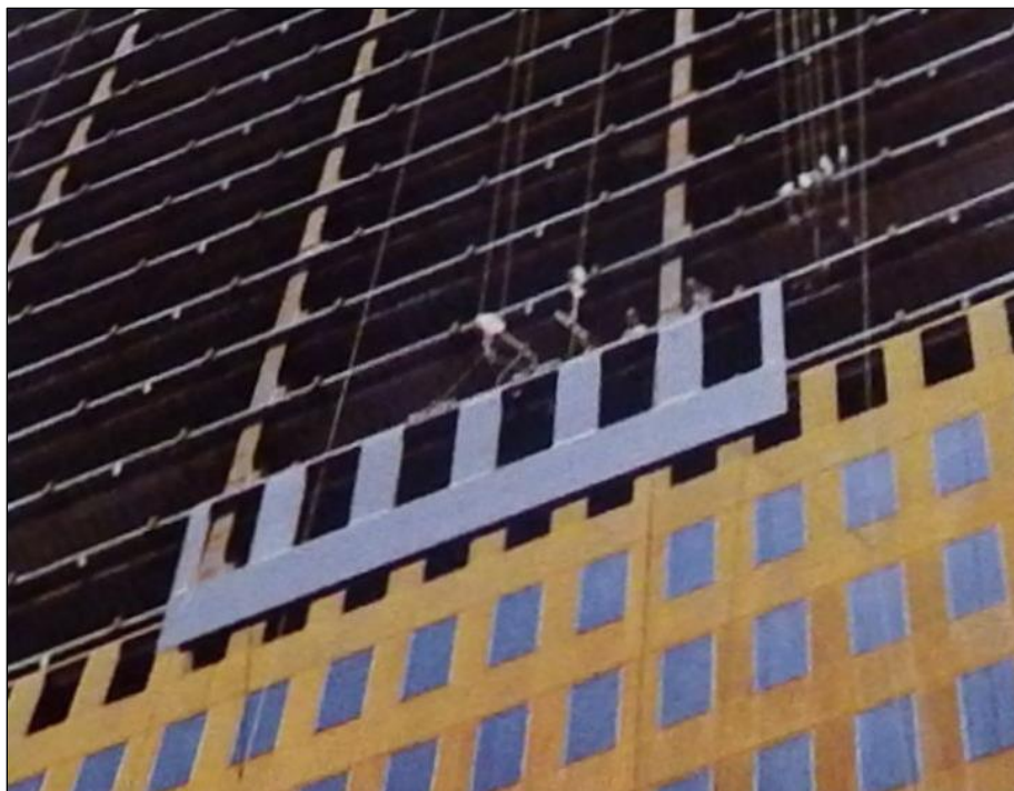
Figure 63: Gray steel panels begin to rust to yellow, orange, brown. ( Mid-West Contractor , July 31, 1974)
