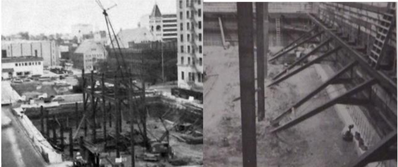
Figure 57: Left, completed excavation, initial steel framing, looking north, right, A-bracing of shoring walls, both ca.mid-1973 ( Mid-West Contractor , July 31, 1974)
