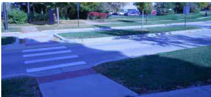
A pedestrian refuge island allows a pedestrian to cross one direction of traffic at a time.
