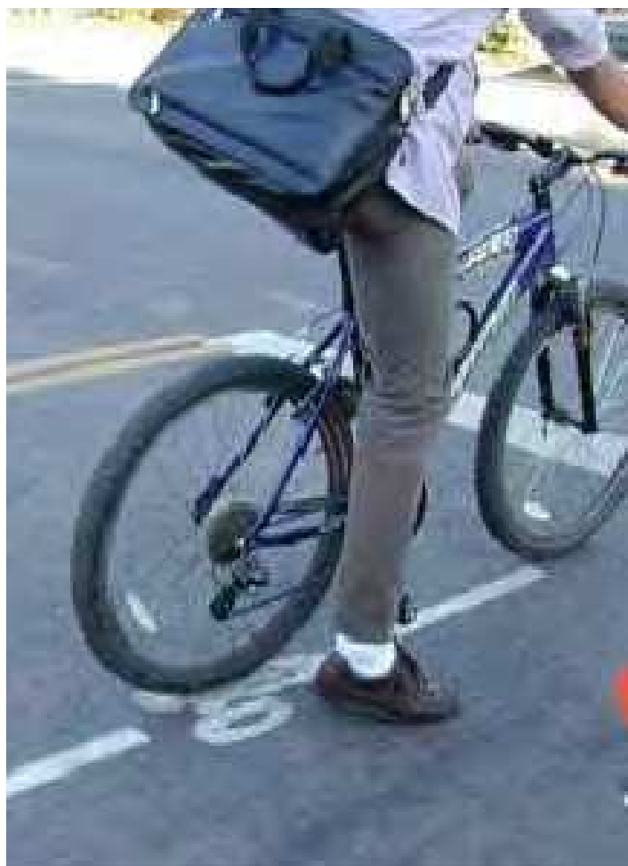
Bike detector markings can be placed at intersections to tell riders where to line up to trigger the signal detectors.
